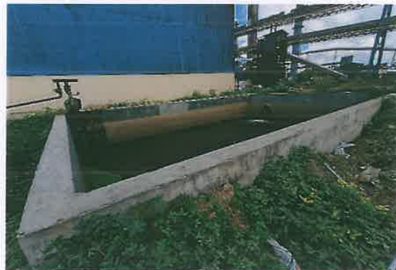
450 m3 Collection tank and pumps arranged at the back of warehouse no. 3
