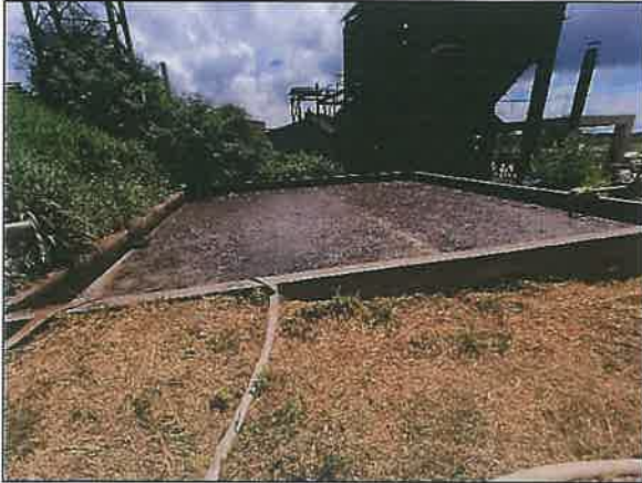
200 m 3 Capacity collection tank provided at distillery for collecting contaminated water
