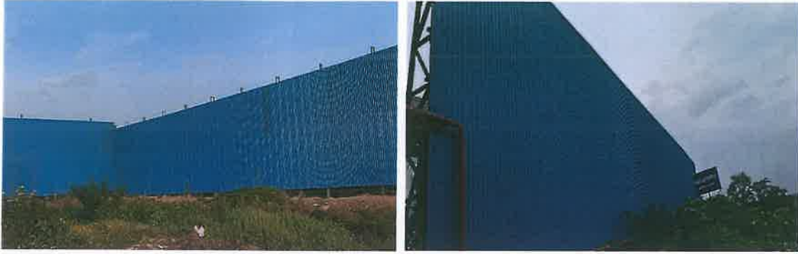
6-Meter-high Barricading provided around the Bagasse yard to avoid fugitive emissions
