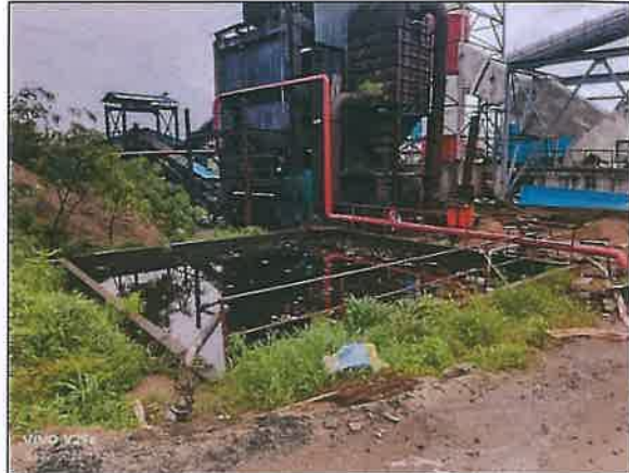
200 m 3 Capacity collection tank provided at distillery for collecting contaminated water
