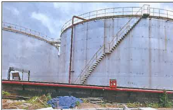
Secondary Containment Dyke wall with control valves provided for the Molasses storage tanks to contain any leaks and to avoid contamination to Hanumantha Pond.
