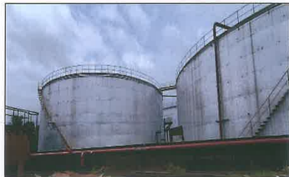
Secondary Containment Dyke wall with control valves provided for the Molasses storage tanks to contain any leaks and to avoid contamination to Hanumantha Pond.
